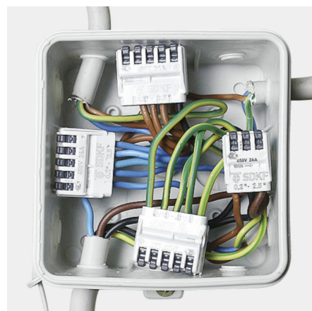
Control window for correctly stripped and pushed-in wires
